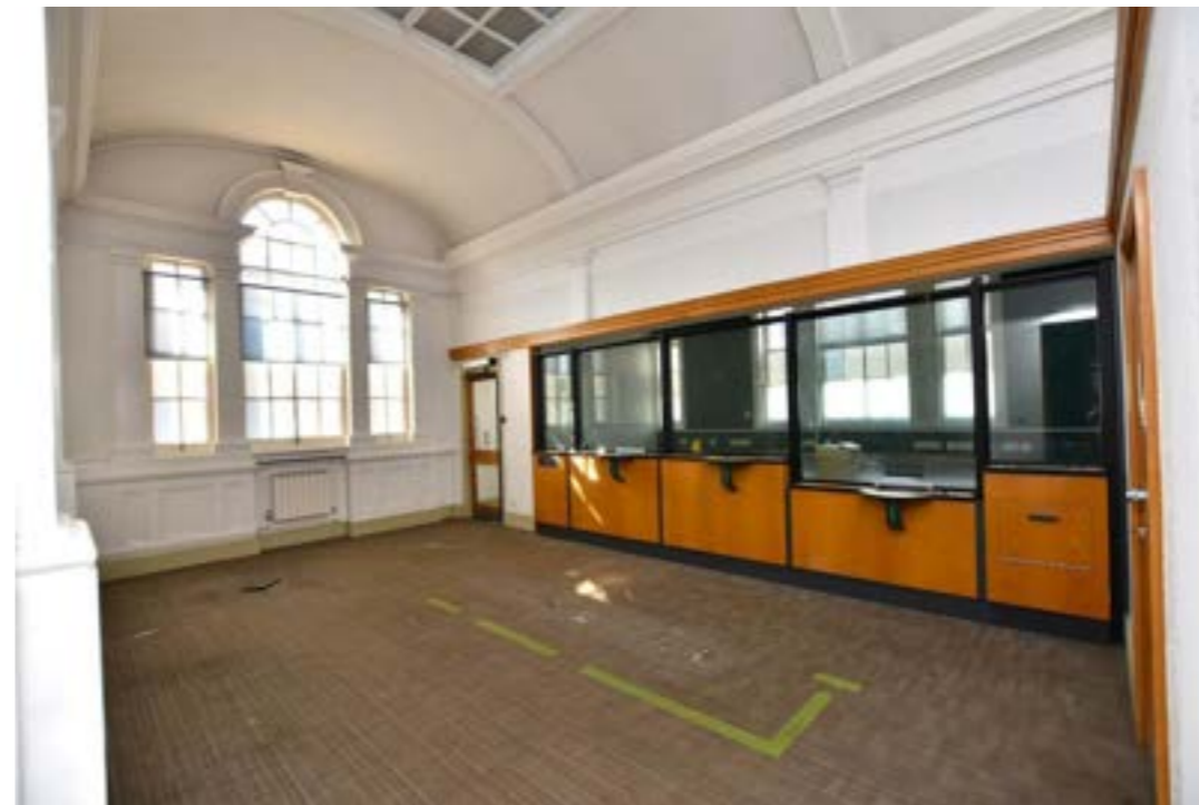
← Internal image of the Grade II Listed bank building
